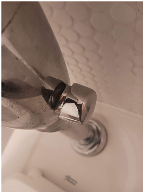
smith library bathroom
